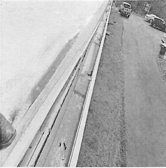
fasteners have deteriorated
